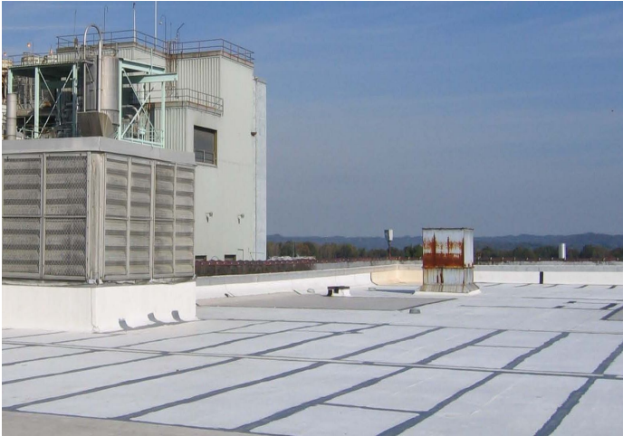
Prepared Single Ply Seams w / SEBS Mastic
